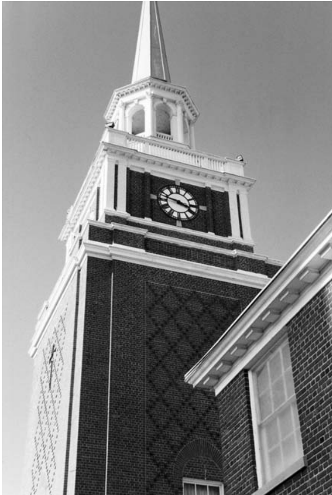
Figure 9. The tower of the Charleston Baptist Temple.
