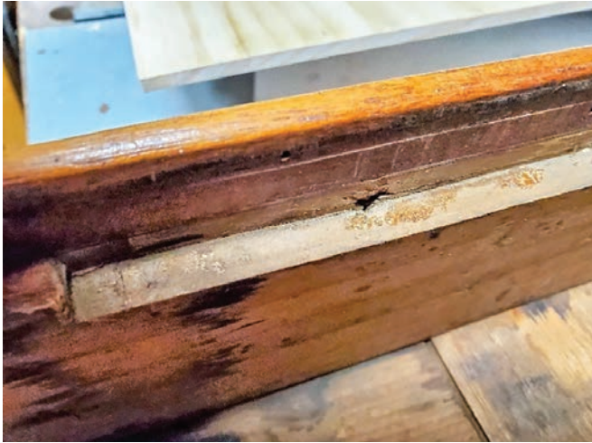
Figure 7. A closer photo of dial relief cut into the case sides, as also seen in Snowden’s example. AUTHOR’S PHOTO.
