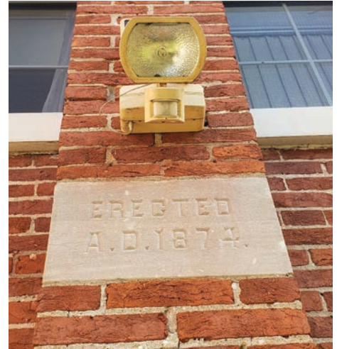
Figure 2C. The original Adams & Perry factory cornerstone with the date of "A.D. 1874" can be viewed today. PHOTO BY THOMAS CUNROD.
