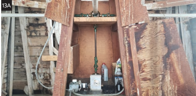
Figure 13A. The electric clock mechanisms that now reside in the East Tower. It appears Hamilton reused the wooden cases of the mechanical clocks, which protected the movement from the environment of the tower. PHOTO BY MELONIE MURRAY. B. The West Tower electric clock was installed in 1940 as a replacement for the clock sent to Thaddeus Stevens College. This clock currently does not work. PHOTO BY TOM CUNROD.
