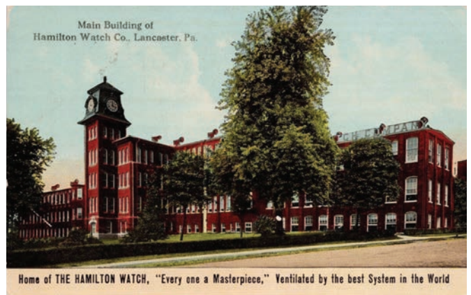
Figure 6. Here is a ca. 1909 view of the factory illustrating the new East Tower featuring a bumped-out center section and more fourth-floor additions. The first clock installed was a Seth Thomas no. 6 tower clock with electric winding. The clock boasted four 6' diameter illuminated dials. COURTESY OF GEORGE MEYER.
