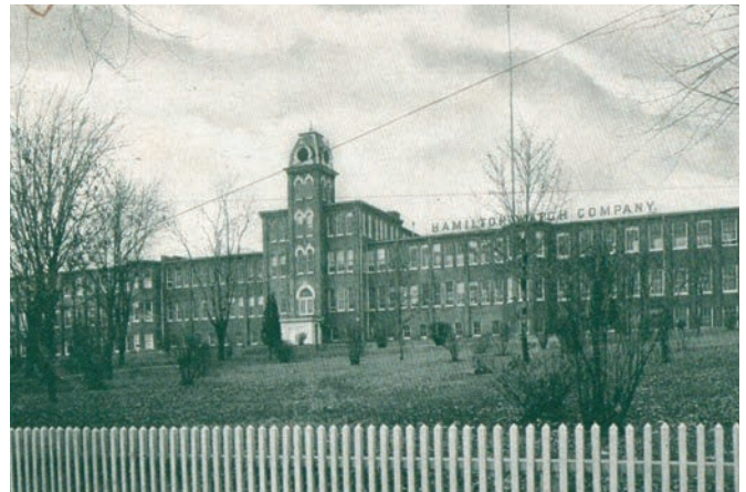
Figure 5. A ca. 1905 photo shows a fourth floor added to the original building, as well as extensions of the east and west wings. COURTESY OF GEORGE MEYER.
