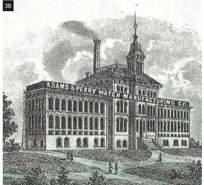
Figure 3A. Pictured here is an engraved image of the original Adams & Perry factory designed by Clarence L. Styles, opened in June 1875. It has been published many times and was accepted as showing what the factory looked like. However, the clock face and wing end cupolas are drawn but were never installed due to shortfalls in capital. A drawing or engraving may not be reliable in showing what a building actually looked like. COURTESY OF GEORGE MEYER. B. This is the engraved image of the factory used on the stock certificates issued by Adams & Perry. There was no factory built at this time so in its absence the company used a modified engraved image of the Cornell factory. COURTESY OF GEORGE MEYER.
