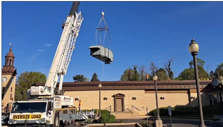
The old air handler was removed in April 2025.
