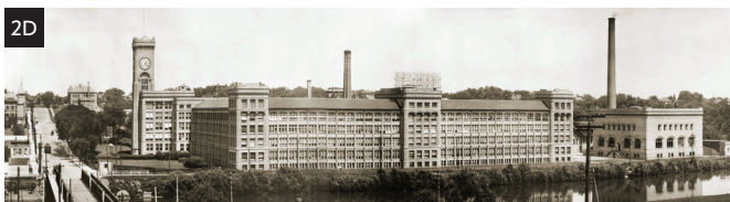
Figure 2A. The Elgin watch factory in 1866. B. The expanded factory in 1868. C. More expansion in 1887. D. The factory ca. 1910, when it was nearly at its largest size and after the front and west (i.e., riverside) sections had been rebuilt. PHOTOS COURTESY OF THE ELGIN HISTORY MUSEUM.
